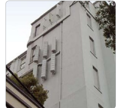
Antennas colour matched and flush mounted to an existing building.
