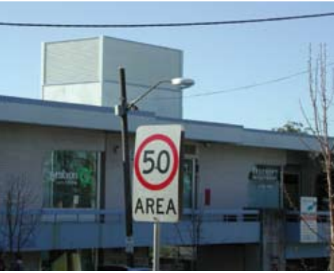
Housing used to screen antennas, cabling and equipment cabin.
