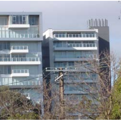
Where multiple Carriers are co-siting, establish a consistent overall height alignment and colour of antennas.
