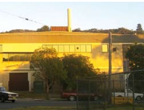
Shroud antennas so that they appear as a chimney or exhaust stack.
