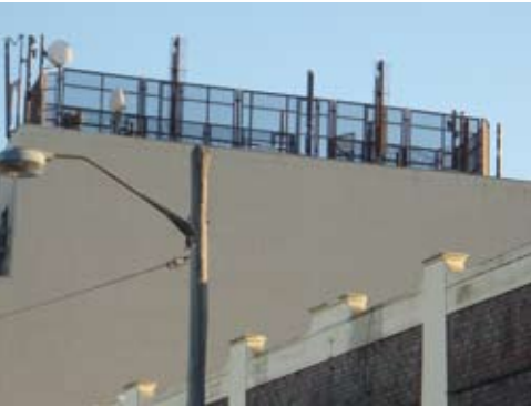
Backscreening can reduce the visual clutter of multiple antennas when placed in relation to primary viewpoints.
