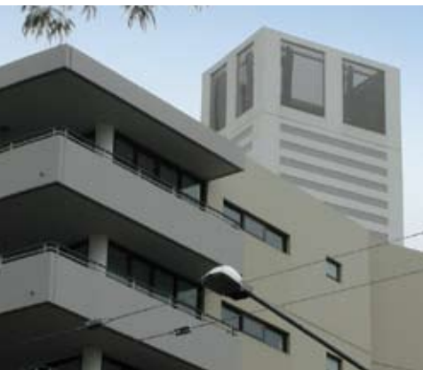
Installing translucent screening can reduce the visibility of antennas against the skyline.
