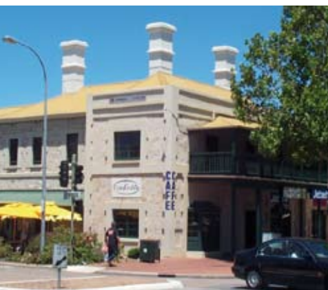
Where appropriate use creative design solutions to screen antennas. in this example, an additional chimney was created on a heritage building.
