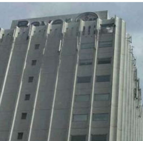
The common alignment of multiple antennas and consistent colour matching produces a better visual effect.
