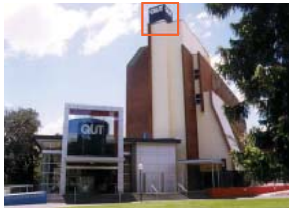
Here, the antennas are within the rooftop signage.
