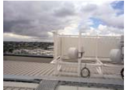
Rooftop screening shown from behind the facility.
