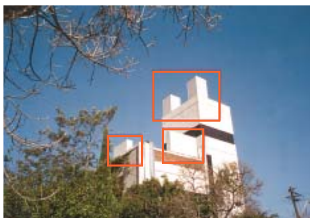
The form and bulk of the original building is blocky and massive. Screening elements can be made to look like part of the original building.
