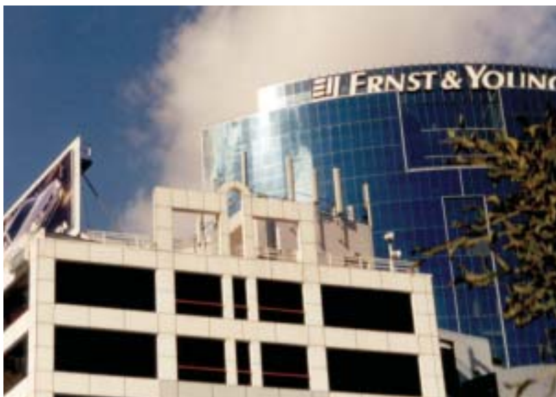
Low-impact CBD rooftop installation
