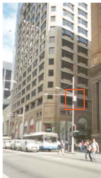
Microcell on a CBD "smartpole".
