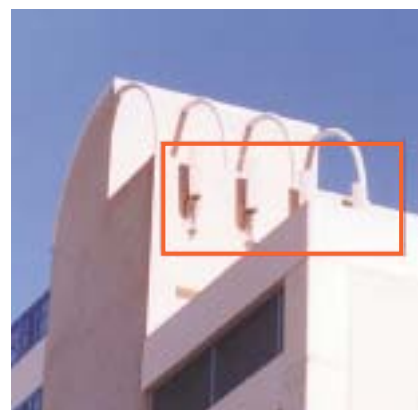
The placement of antennas in this example emphasises the form of the roof.
