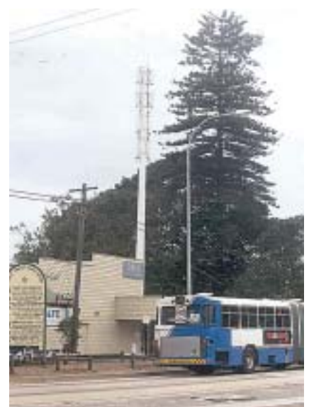
It may be inappropriate to use a bulky headframe if co-locating on this pole.
