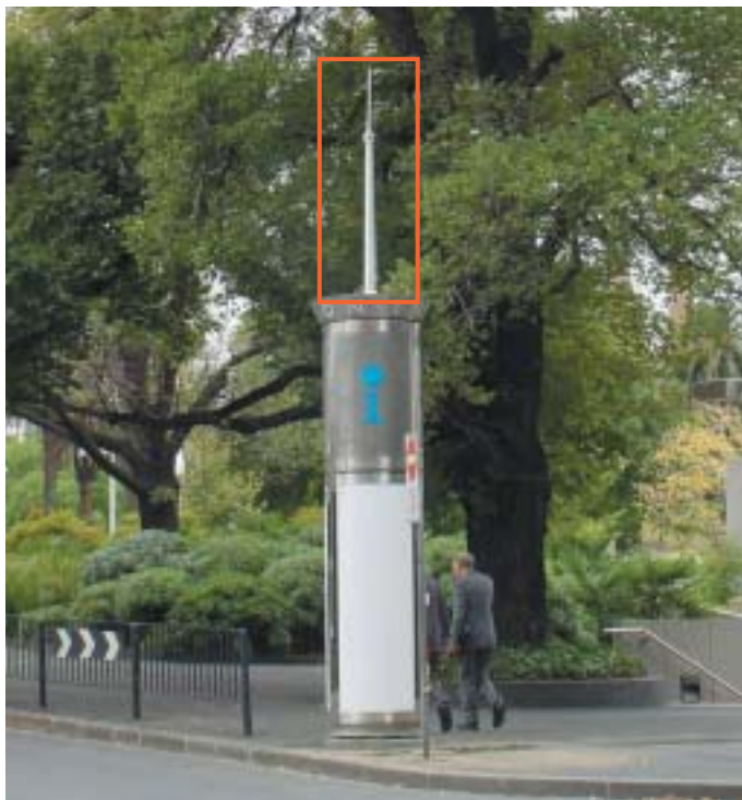
A colour matched patch antenna. Here is an example of how an antenna has been well placed and designed, in the context of an important view.
