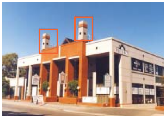
Antennas are located within the column elements in this example.
