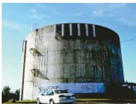
Co-location on a water tank
