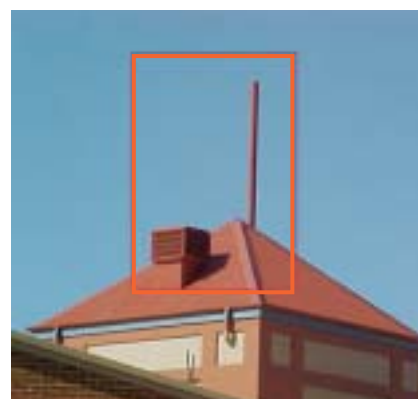
The engineering design of this facility allowed the antenna to be constructed as the "mast" and the dish to be placed within the "air conditioning unit".
