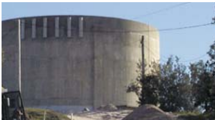
This example demonstrates an ordered approach to the placement of antennas to reduce clutter while fulfilling the site's radio requirements.
