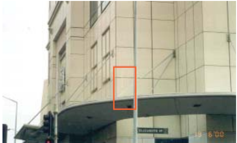
An awning mounted colour matched whip antenna.
