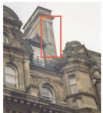
Antenna matched to the stone background.
