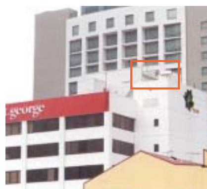
Rooftop cabins integrated with the colour and form of the building. Note also the colour matched antenna.
