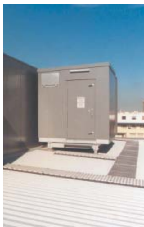
Low-impact prefabricated equipment cabin.
