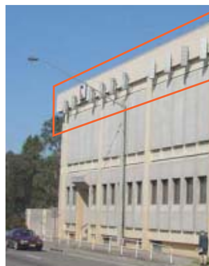
The placement of antennas here repeats the pattern of the windows below.
