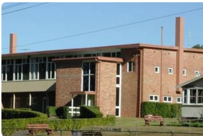
Legal action was needed to resolve this site dispute. Antennas are masked in the two false chimneys.
