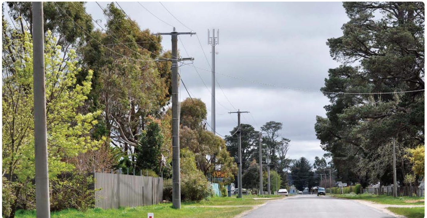
A photo of the proposed base station in Romsey. The base station in the photo is an artists impression of what the tower will look like.
